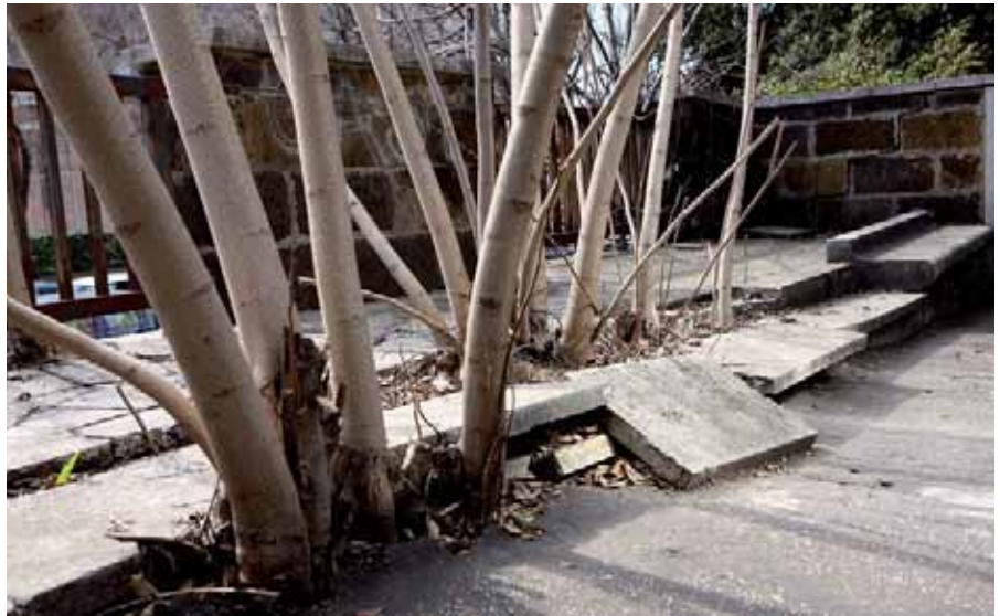
Ailanthus altissima , whose roots inflict serious damage on man-made constructions. Photo J. Grapow
